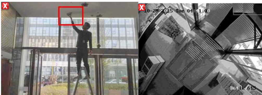
Passenger flow in slant direction (wrong)
